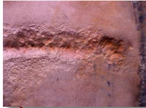
Water Flow Erosion 7 mm Plate
